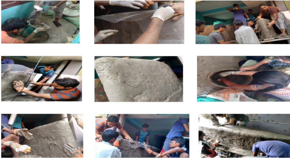
Figure 1.1. Casting of the concrete in the mould
